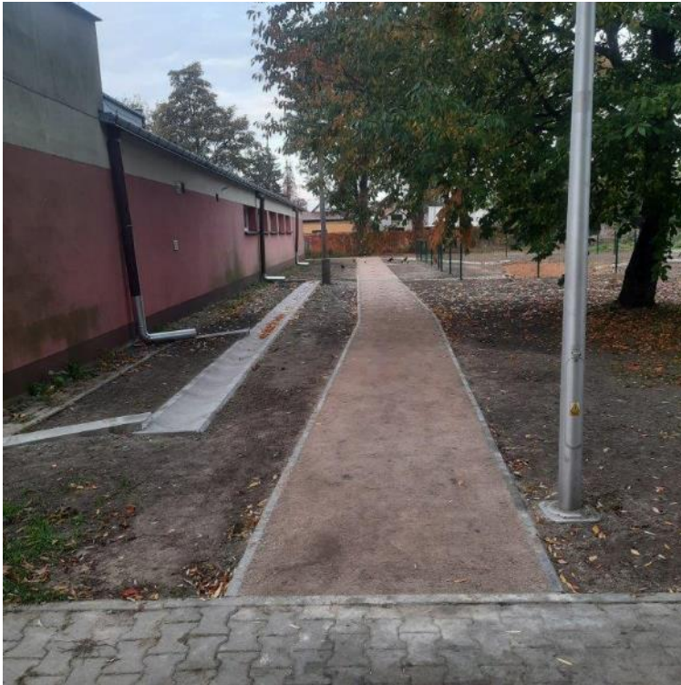
Photo 6 Appearance of the site after construction – Permeable surface
