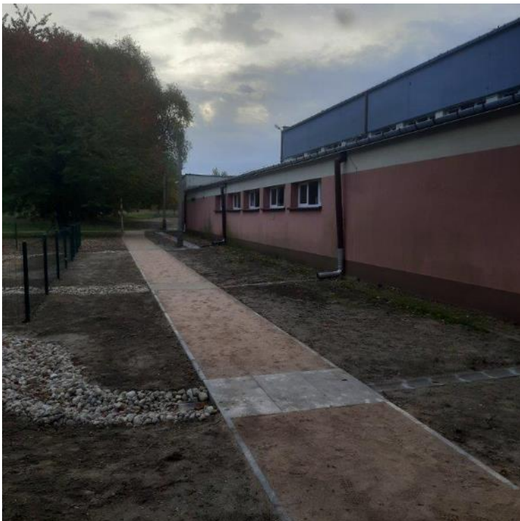
Photo 7 Appearance of the site after construction – Permeable surface
