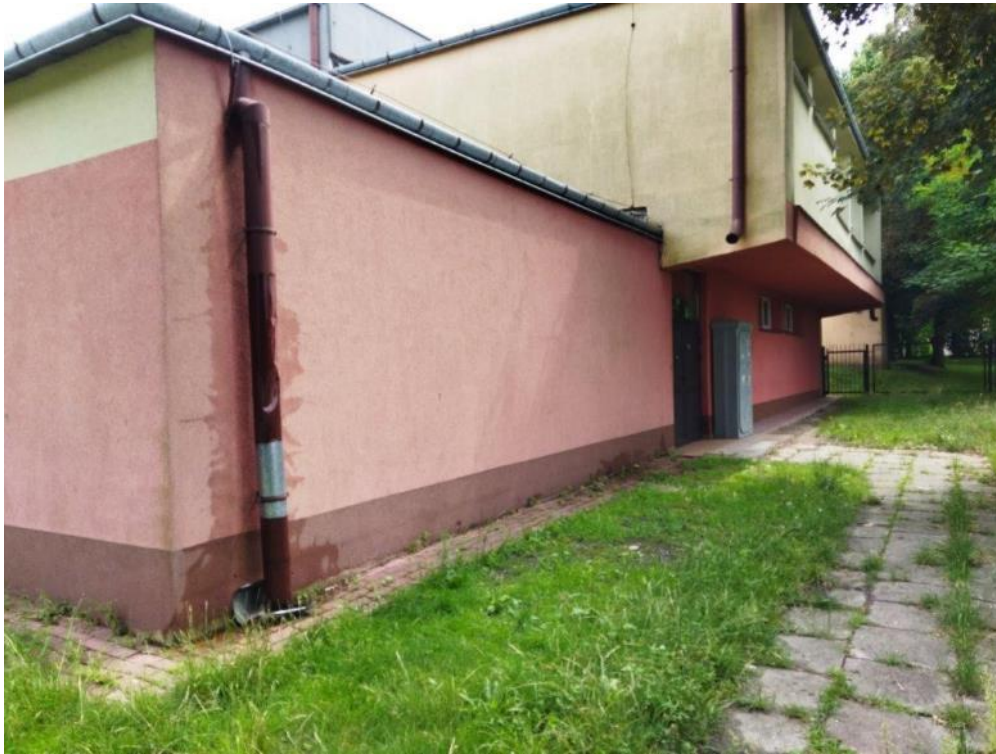
Photo 1 Appearance of the site before construction - Rainwater tank and Permeable surface
