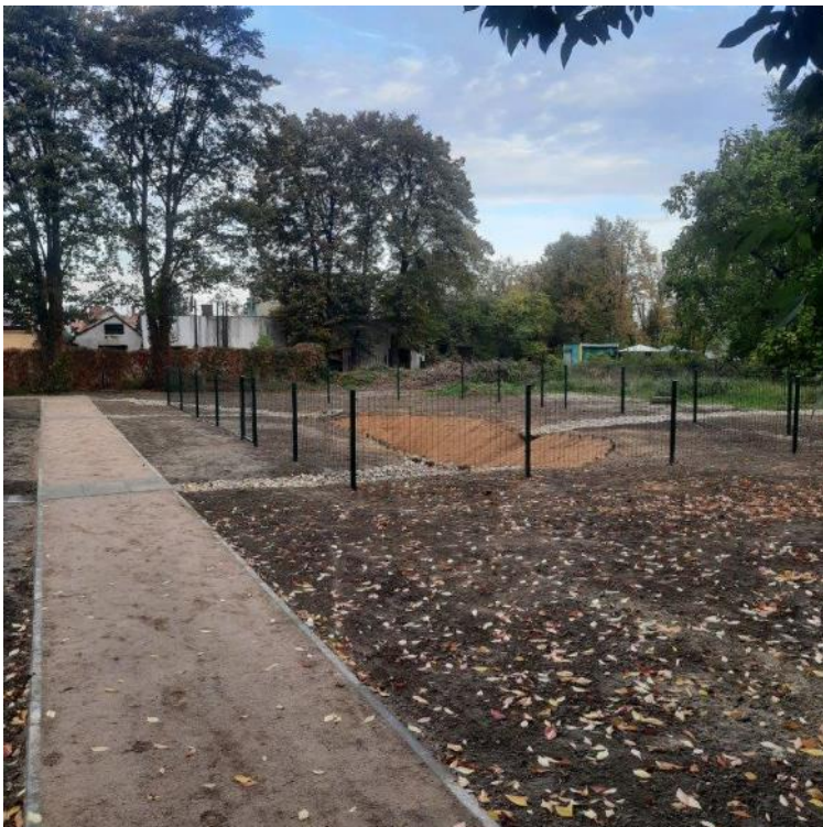
Photo 9 Appearance of the site after construction – Permeable surface
