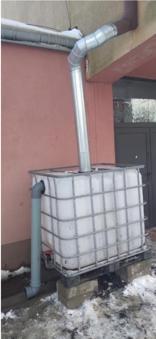
Photo 5 Appearance of the area after construction – rainwater tank
