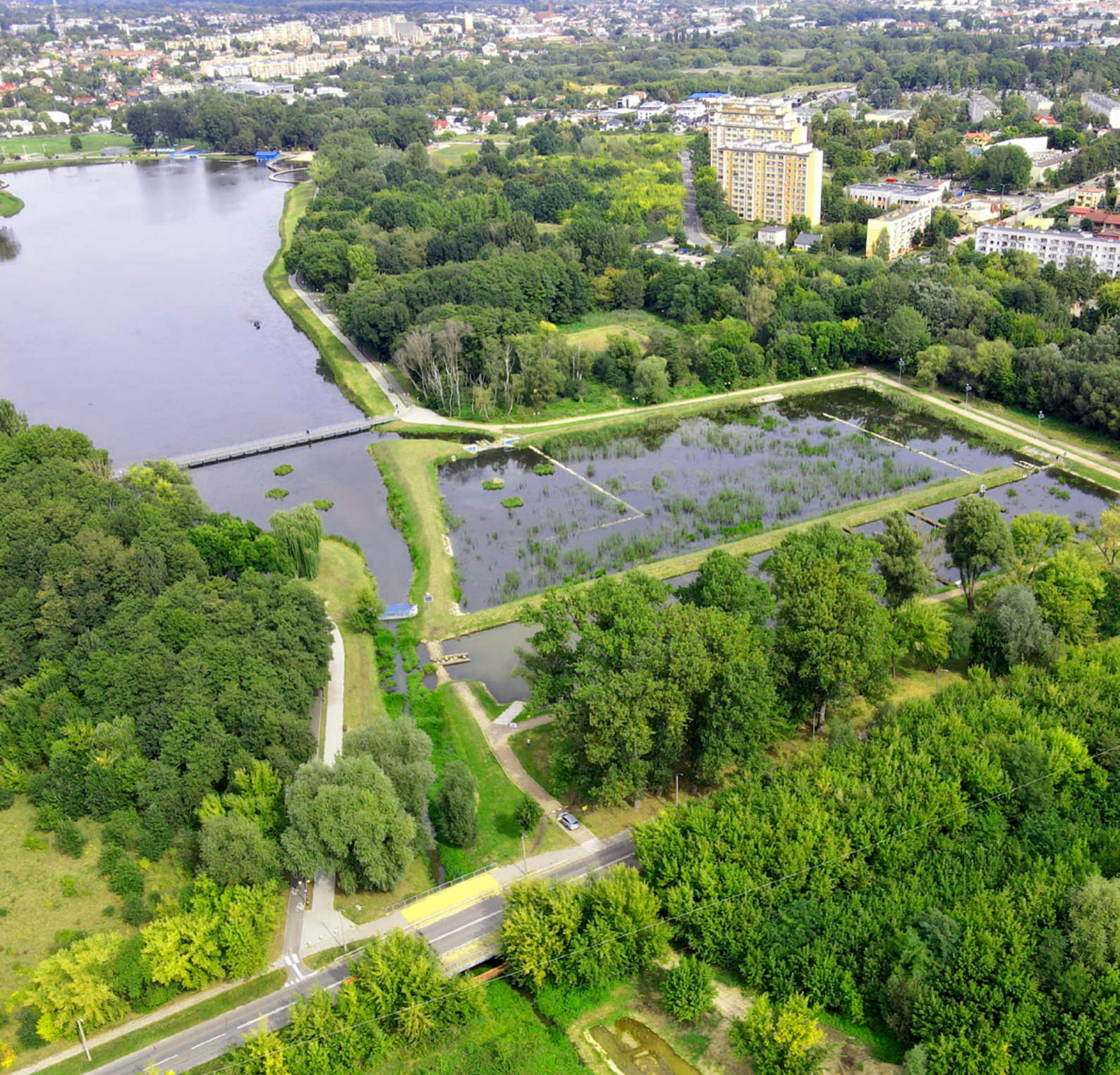
Borki reservoir and colmatation ponds
